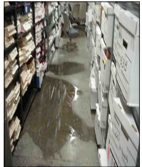
The Lane Construction Company's archives department showing evidence of the sewage loss we faced upon entering the building.
