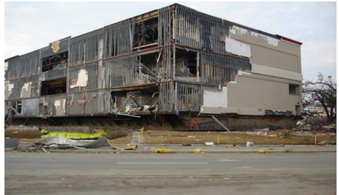
“Floating casino that broke away in Biloxi, MS” (note the bottom hull structure)
